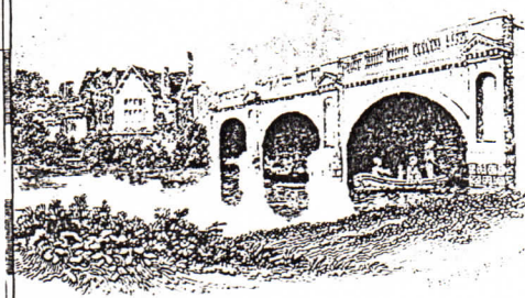
ST. MARY'S BRIDGE AND CHAPEL, DERBY
